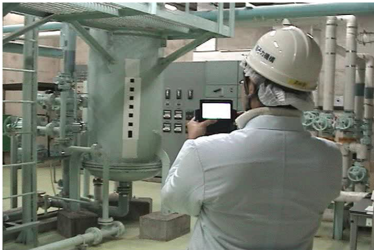
Target: Ion Tank of Pure Water Facility
