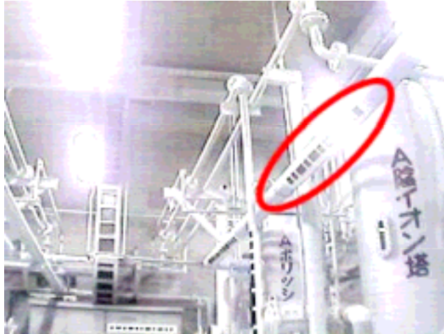
Figure 9: A Case When a Marker Image was Captured against Light.
